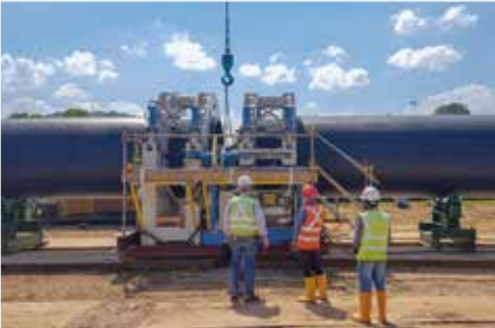
SITE BUTT WELDING EQUIPMENT FOR PIPES AND FITTINGS UP TO OD 3500 MM
